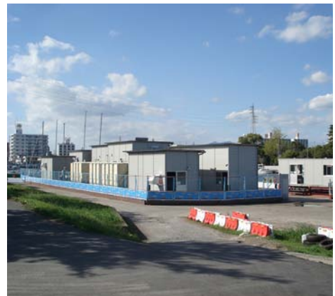
Water purification facility at Tsuchiura Port
