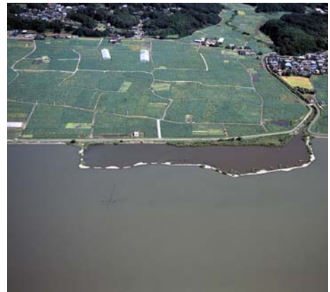
Wetland constructed at the mouth of the Kawajiri River
