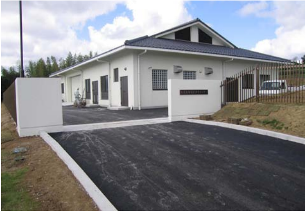
Namegata City Tamatsukuri North Regional Wastewater Treatment Plant (appearance)
